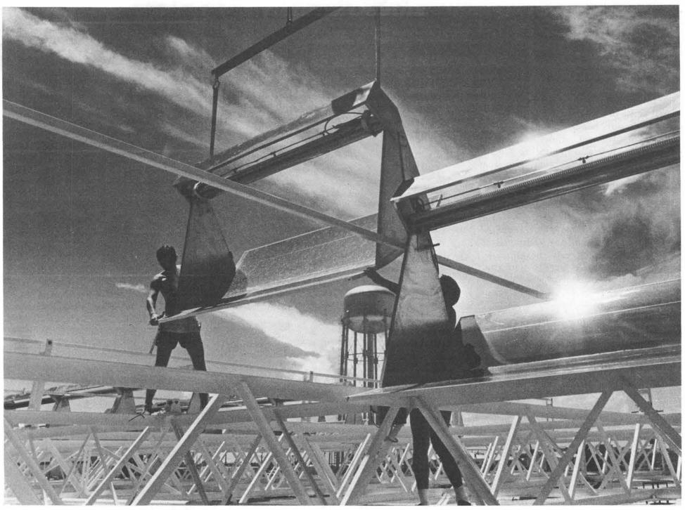
PHOTOVOLTAICS ADVANCED SYSTEMS TEST FACILITY is now open for business. Located just northeast of the geodesic dome (Visitor Center), the facility is newest of Labs' solar installations and is dedicated to testing of photovoltaic arrays—devices which can convert solar energy directly into
